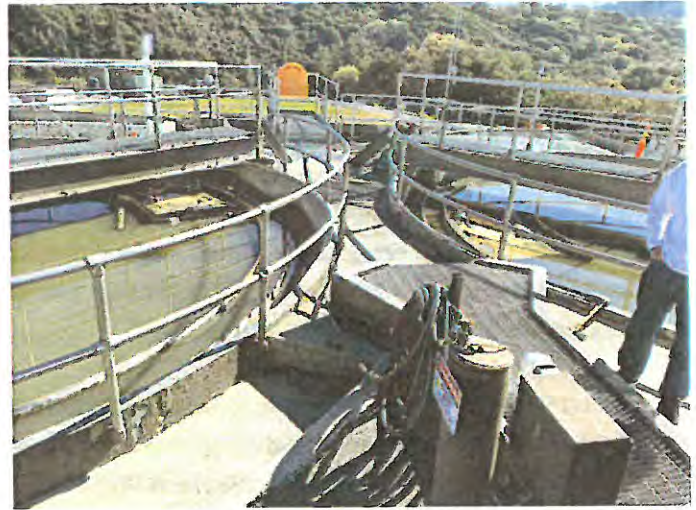
Figure 1. Existing Primary Clarifiers
