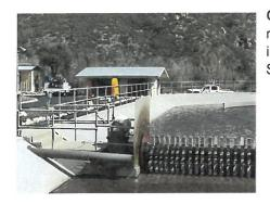
Cleghorn Treatment Plant – Standby generator (equipment starts automatically) runs on propane (1000-gallon tank). Test run twice a month. Scheduling for inspection of generator and transfer switch by in-house Electro-Mechanical-Specialist and District Mechanic. Propane tank will be filled as necessary.
