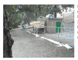
Lake Gregory Lift Station – Generac, diesel fueled standby generator. (It is critical this lift station never fails. A spill here, is into Lake 'Gregory). Maintenance staff has installed appropriate connections needed to utilize the 2000-gallon tanker to manually haul from this station in an emergency. Each load taken to the Huston Plant influent interceptor requires approximately 45 minutes. Thompson Pump equipped to run bypass to empty wet well when needed.
