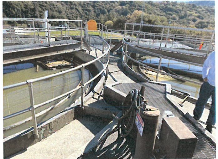
Figure 1. Existing Primary Clarifiers
