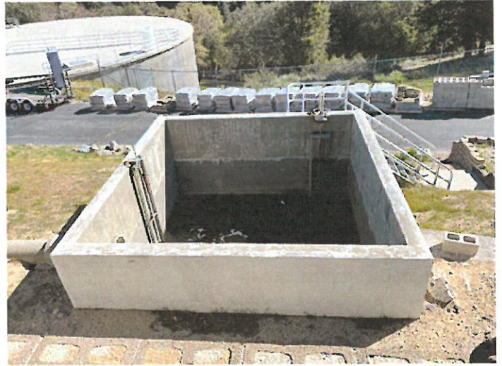
Figure 5. Existing Diversion Box to Emergency Storage Reservoir
